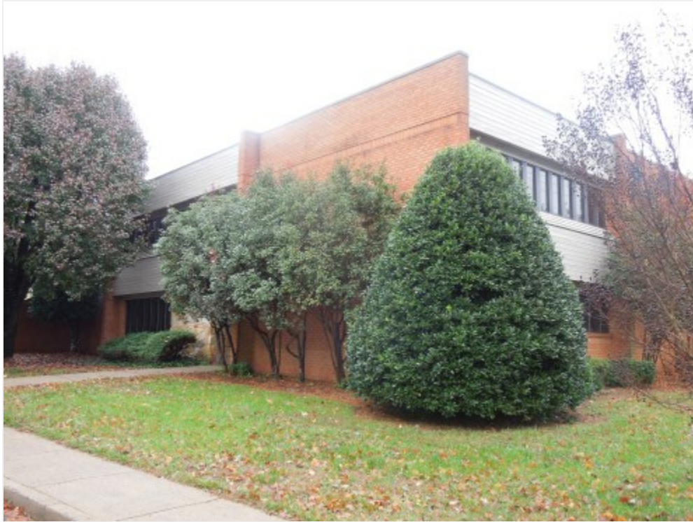
Space is on ground floor
